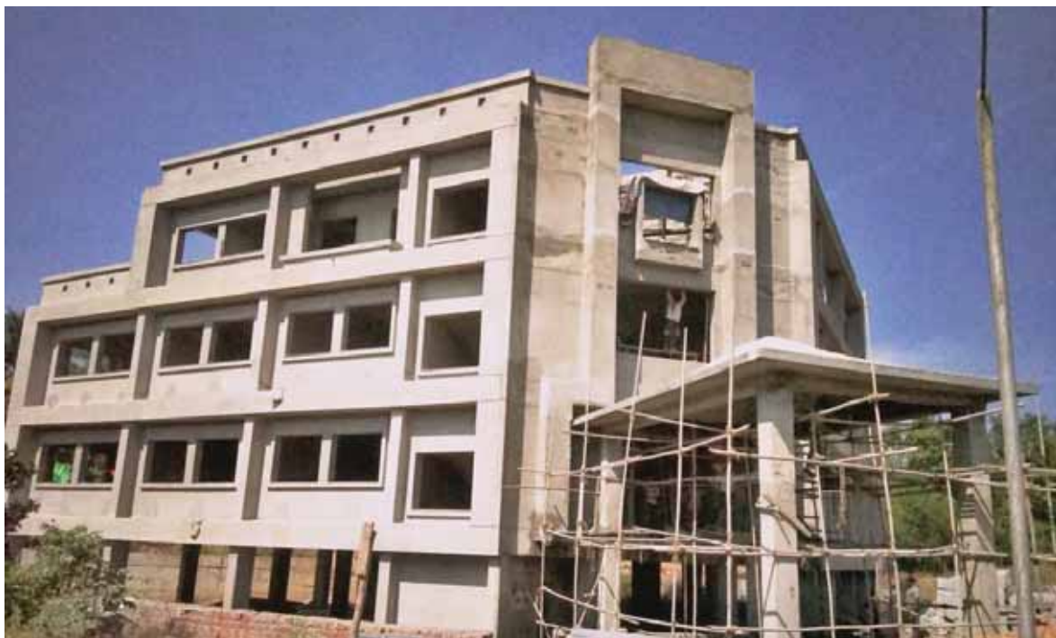
JSS Resource Centre, Sindhudurg
